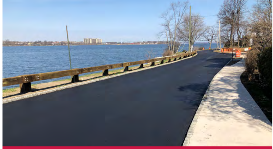
Green Asphalt paved Shore Road in Queens in New York City with its 100-percent recycled asphalt product. Photos courtesy of Green Asphalt.
