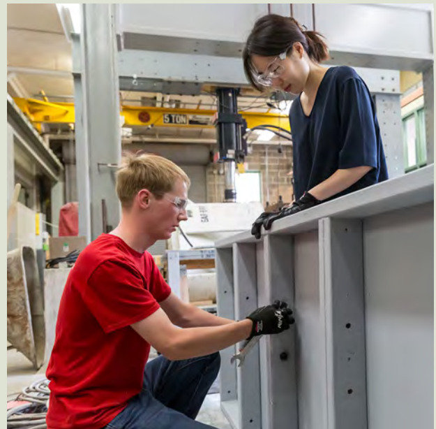
Undergraduate Lennart-Fredrick Schmitz and postdoc Hyeyoung Koh build a vacuum box in the Jun and Sandy Lee Wisconsin Structures and Materials Testing Laboratory. Assistant Professor Hannah Blum will use the vacuum box to test steel decks and other structures. Photo: Alex Holloway.
