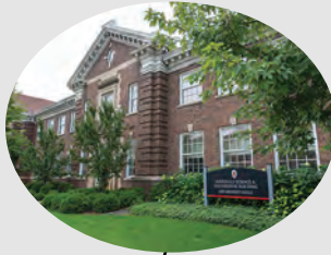
5. MATERIALS SCIENCE & ENGINEERING BUILDING
