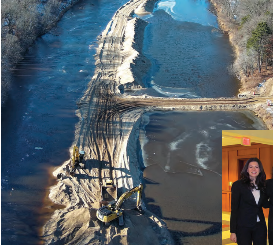
Left: An aerial view of a sand trap dredging operation on the Eau Claire River. The river flows into Lake Altoona, carrying sediment that has caused challenging buildups for the community. Photo courtesy of Eau Claire County. Below: Civil and environmental engineering students Maya Pardanani, Kris Alvarado, Clara Zwolanek, Dylan Schindler and Rachael Heck (from left) worked together on a project to address sand buildup in Lake Altoona in Eau Claire County during the fall 2023 semester. Submitted photo.
